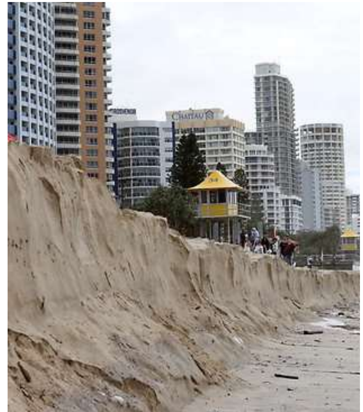
Surfers Paradise Beach has suffered major erosion damage after the coastline has again been hammered by large swells. Picture: Adam Head, The Courier Mail Feb 23, 2013
